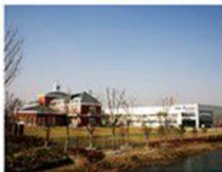
昆山美国工业村综合维修厂 Kanshan Eastern American Industrial Village
